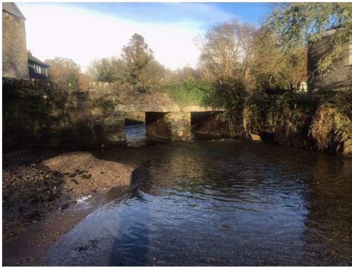
Lower Penpol Bridge
